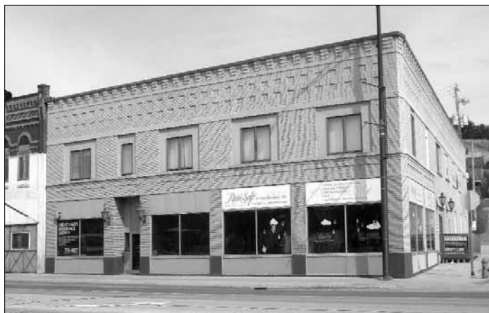
The Kingsford Motor Car Company building as it appears today. It is divided into small business spaces. Photo by Guy Forstrom.
